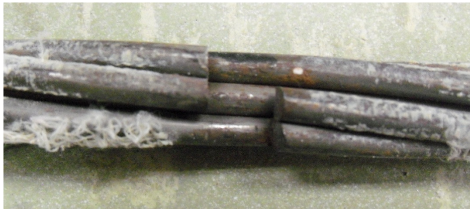
Figure 5.21 The 7-wire strand with two-broken-wire defect.
