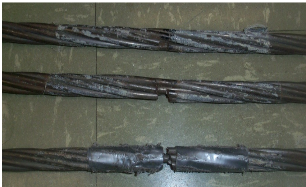
Figure 3.10 Typical steel strands with bundle of wires used in main cables of cable-stayed bridge; Showing man-made defects, from top to bottom, of one broken wire, two broken wires and five broken wires.
